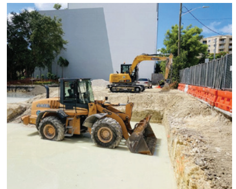
Construction site. Photo: Raychel Lean/ALM
